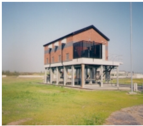
Fig 4 Preston WwTW UV plant
