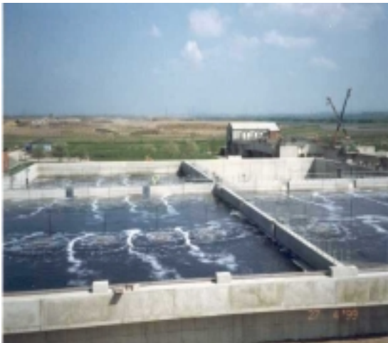
Fig 3 Preston WwTW storm tanks
