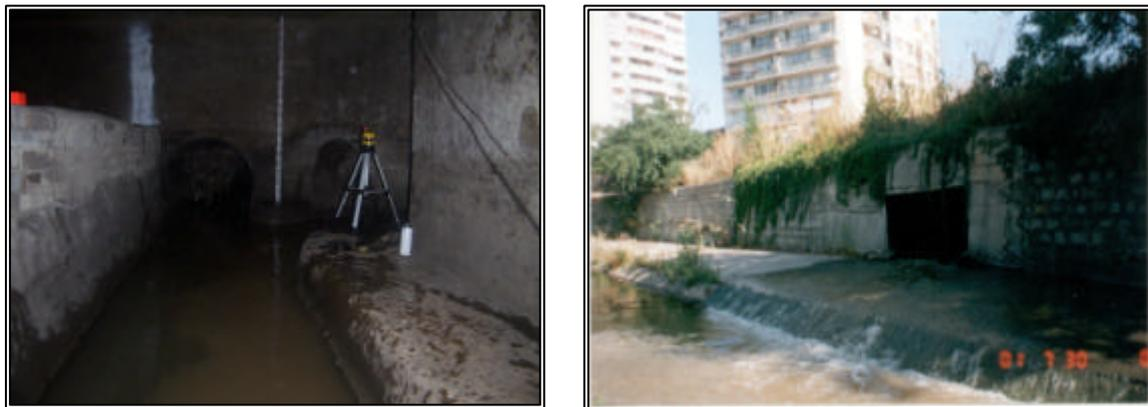
**Photograph 1: Photographs of a CSO internally and spilling to the river Suhodol in dry weather.**
