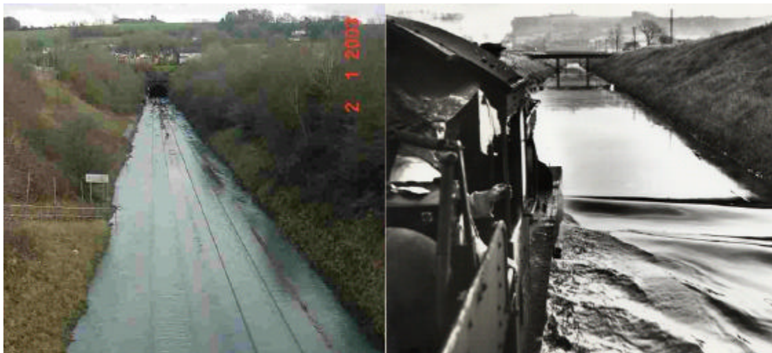
Figure 2 – Modern Day Flooding and a Steam Engine Passing through Flood Waters (Both West Cutting Looking East)
