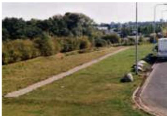
maintenance of the filter strip. There is no evidence of excessive silt accumulation. If the silt loading on the filter strip is assessed the thickness of silt that would theoretically have accumulated over the eight years is about 0.6mm, ie it will not be noticed in a grassed area.
