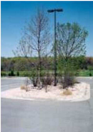
**Figure 6 Bioretention area**
