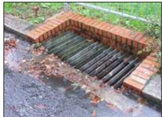
Supergulleys (as shown in the previous photograph) have very large waterway openings and generally measure 1.35m wide by 0.675m deep with a 300mm or 450mm dia outgoing pipe. The size of these supergulleys are such that pedestrian barriers are required around them to protect members of the public. These supergulleys can take very large quantities of water off the highway.
