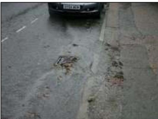
There are of course other factors which can influence the performance of road gulleys including the distance between the gully grating and the kerb, the degree of maintenance, the extent of blinding with leaves or litter, any drop kerbs and local variations in road levels (see photo). To take account of all the factors which influence each individual gully would be far too time-consuming and clearly a more simplified and standardised approach is needed.
