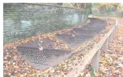
Figure 4 Stepped swale in Keighley
