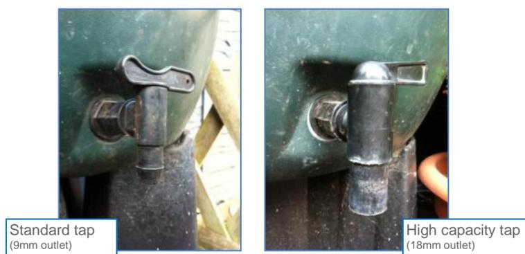
Figure 13 – Types of water butt tap.
