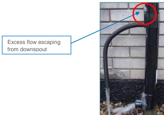
Figure 5 – Photograph showing spill exceedance of the basic diverter.
