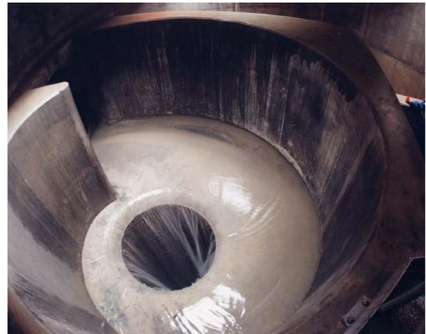
Figure 4 – Example of the scroll type vortex
