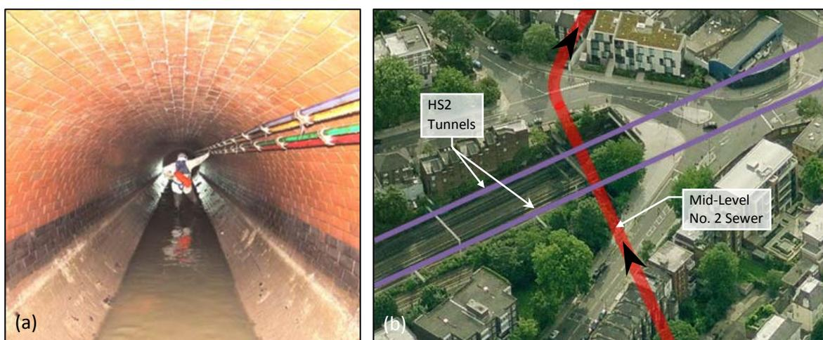
Figure 3 - (a) Recent survey photo inside the Mid-Level No. 2 sewer (Courtesy of TWUL) (b) Plan showing the intersection between the proposed HS2 tunnels and the Mid-Level No. 2 sewer (Bing Maps imagery)
