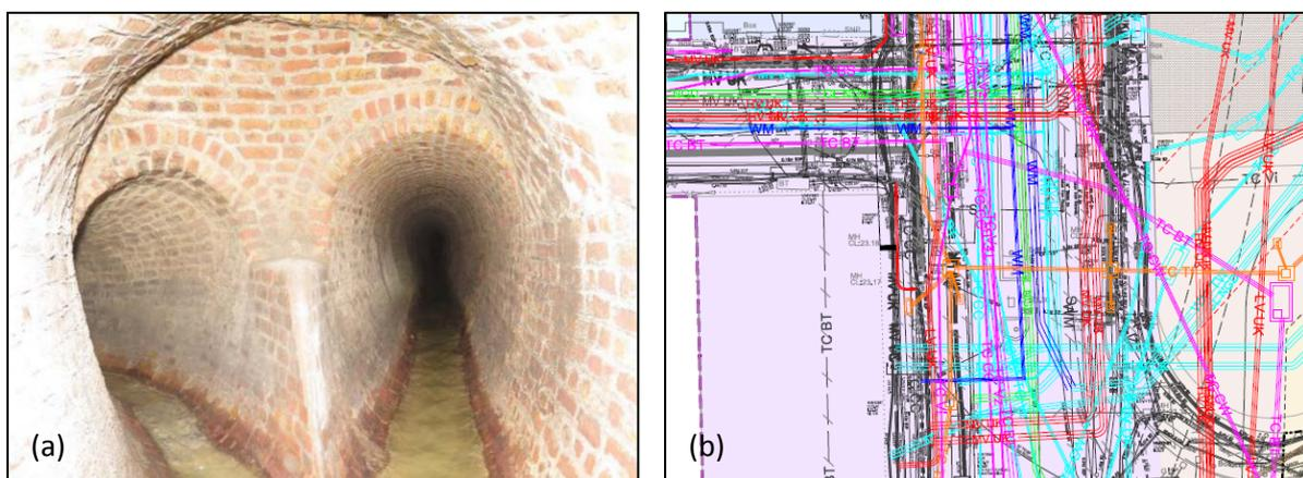
Figure 2 - (a) Typical Central London brick egg sewer junction (courtesy of TWUL) (b) Extract from the proposed Euston Station Combined Utilities Design, showing the complexity of utilities in this area of London (courtesy of HS2)
