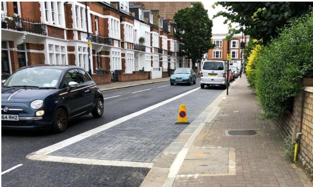
Figure 4 - Example of completed scheme showing permeable pavement and geocellular storage below parking bays
