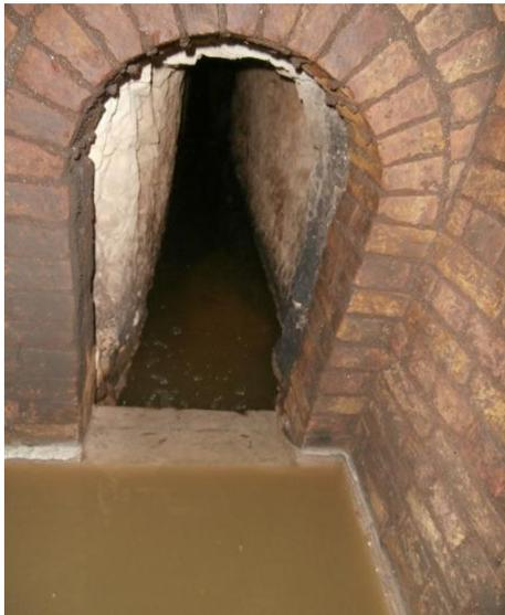
1. physical damage to the sewers (for example broken pipes, failed laterals and joints) within the tunnels allowing sewage to escape
