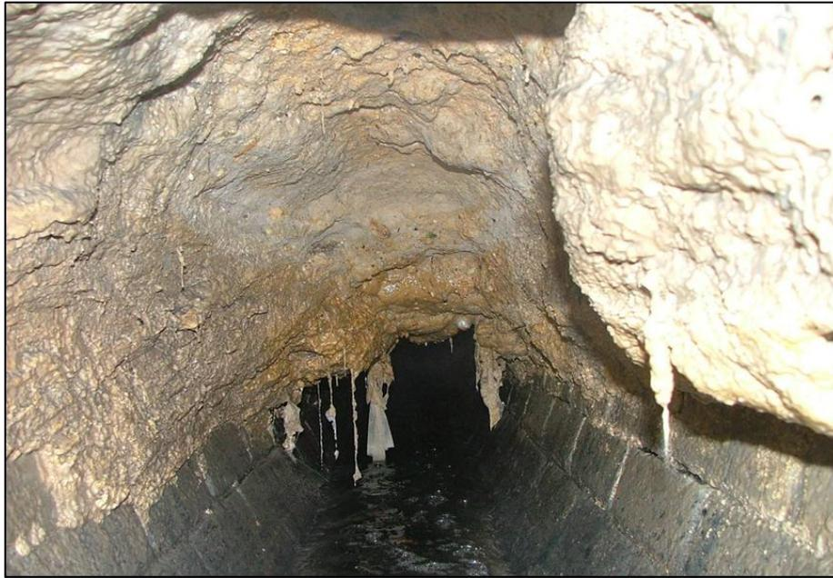
*Significant deposits of FOG fouling large brick sewer*
